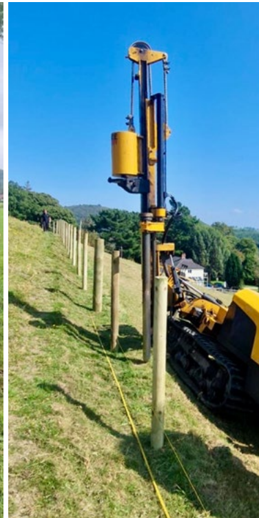
▲ Tidy work erecting a stock fence
