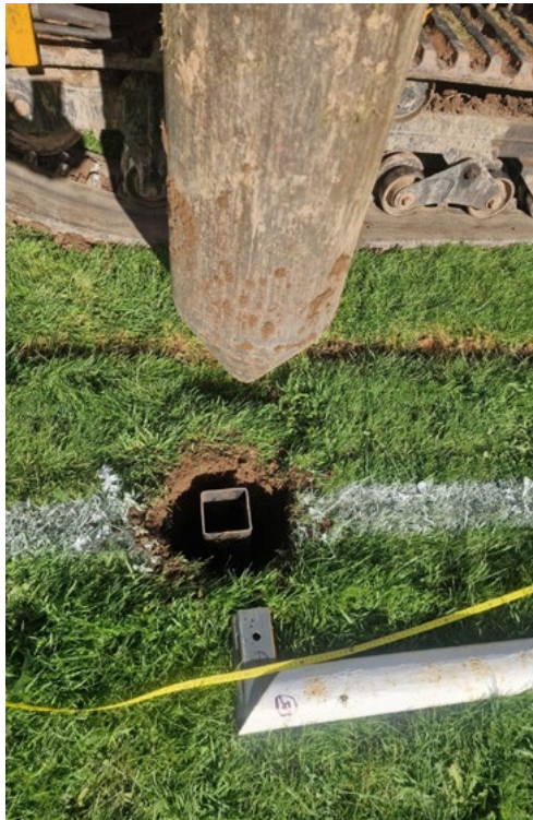
▶ Installing metal sockets
