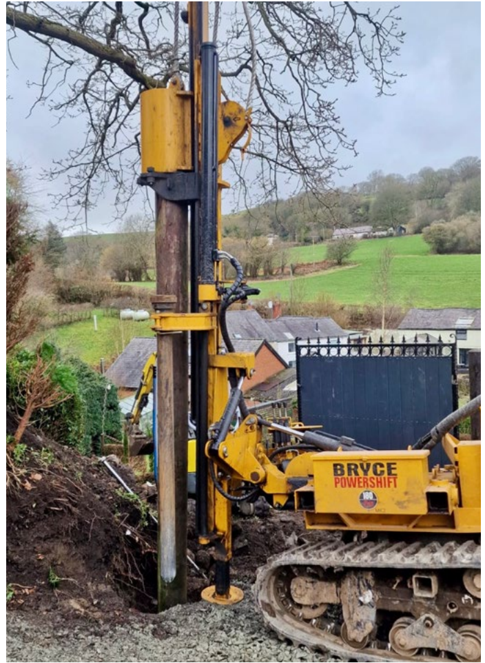
▶ Driving a 3.6 metre post
