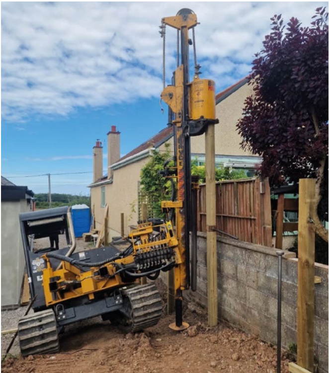
▲ Erecting domestic fencing
