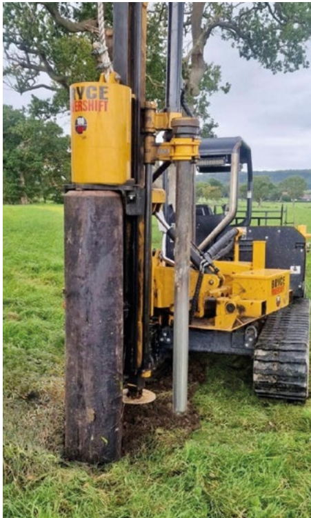
▲ Driving a heavy gate post
