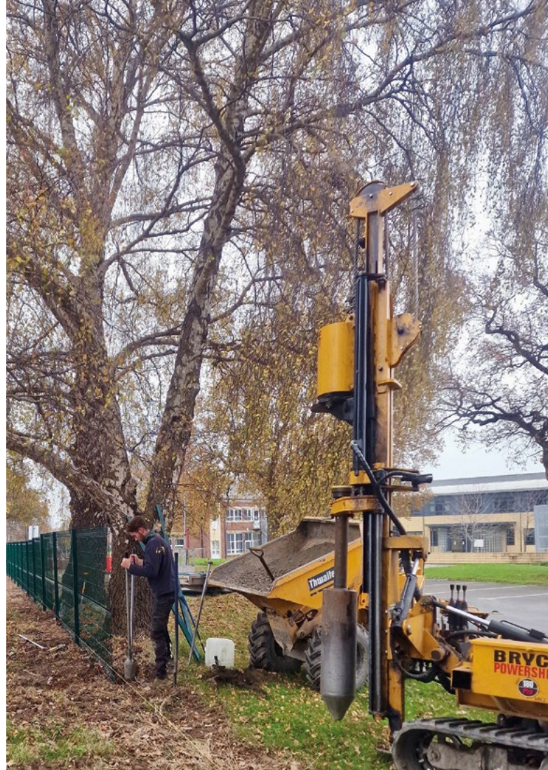
▲ Erecting security fencing
