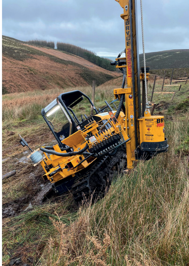
▲ The Bryce 180 PRO debogged itself using Power Slew and Weight Transfer
