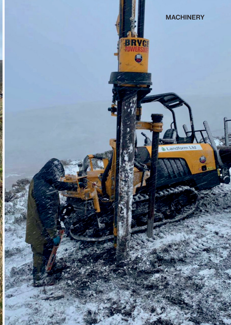
▲ Working high out under adverse conditions
